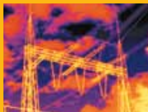
Inspection of high voltage power lines
