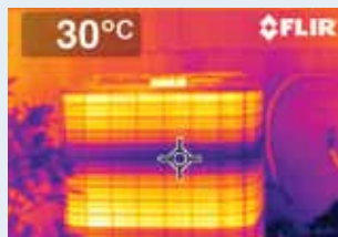
What a thermal imaging camera sees.
